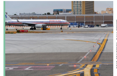
Runway status lights will greatly reduce the possibility of runway incursions and improve safety on LAX runways.
