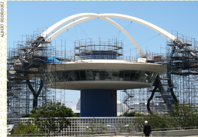
ABOVE: The LAX Theme Building renovation nears completion with new moisture-proof stucco and seismic retrofit.
