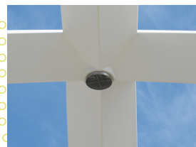
ABOVE: This unique air vent at the pinnacle of the Theme Building will help remove moisture from the interior of the arches.
