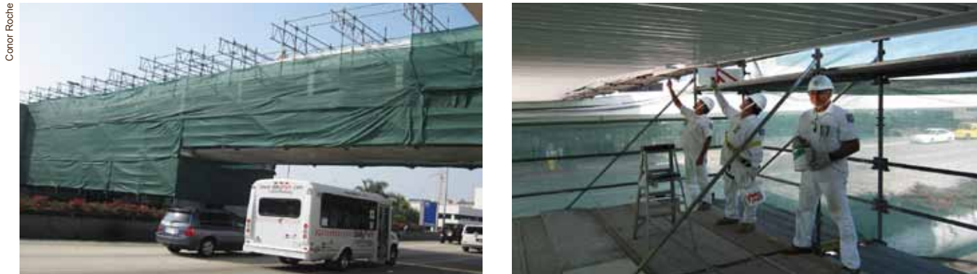
Left: Scaffolding on the pedestrian bridge between Parking Structure 2 and Terminal 2 allowed workers to repaint the structure without inconveniencing passengers and blocking roadways with lift equipment. Right: LAVA Maintenance Service Division personnel paint a side of the pedestrian bridge. (Left to right) Painter Bruce Pugh, Lead Painter Raul Medina, and Painter Hector Cortez.
