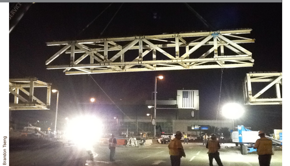
Removal of the pedestrian bridge between Parking Structure 4 and the Tom Bradley International Terminal facilitates construction of the Central Terminal Area Curbside Appeal Project.
