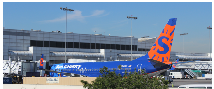
CLOSING THE GAP – Terminal 1.5 is a building that will connect Terminals 1 and 2, and will be located in the current open space between them.
