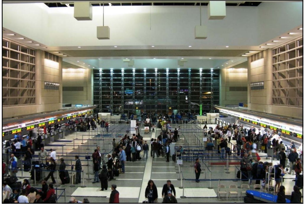
The photo above shows the TBIT Departures Lobby with the new over-ticket counter lighting dimmed 50% on the left side and at full 100% lighting on the right side.
