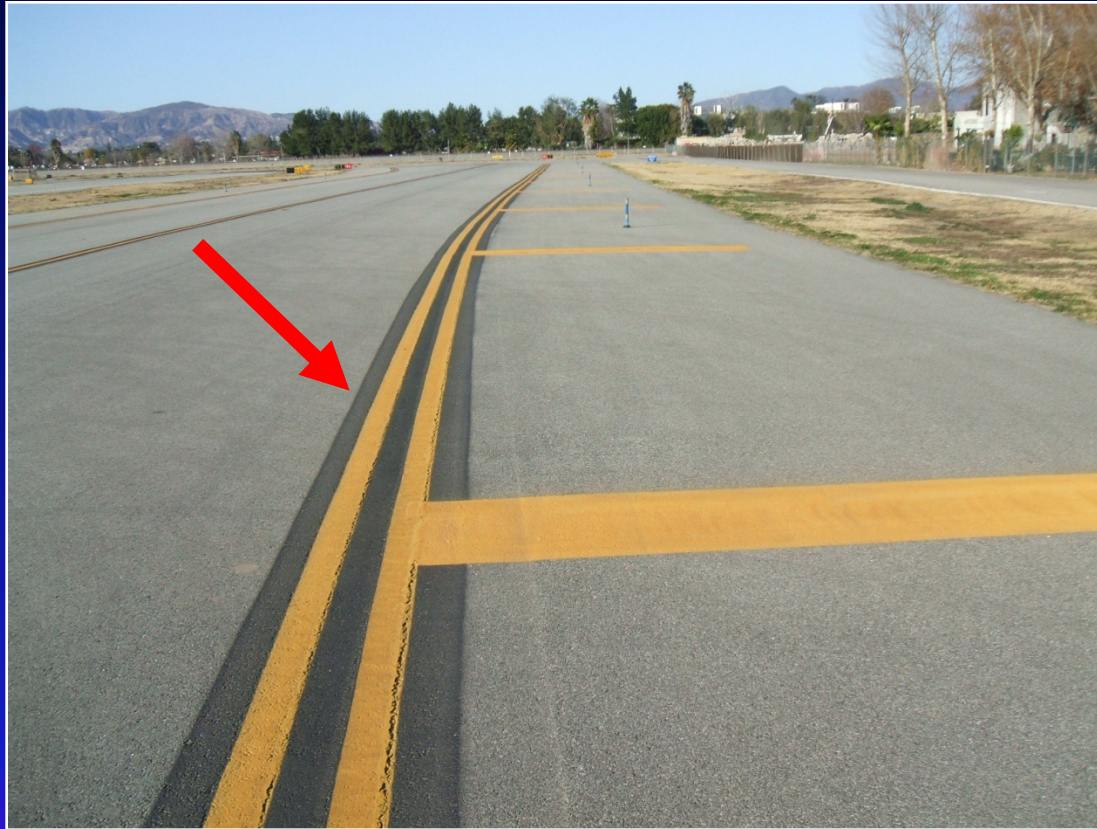
Taxiway Edge-line with Shoulder Markings
