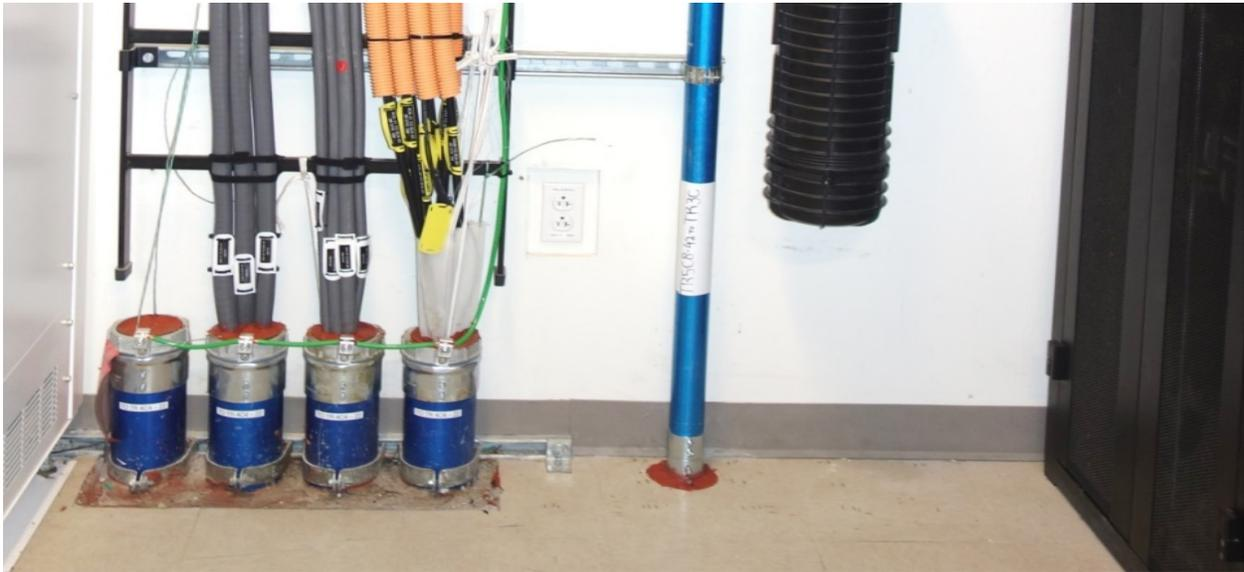
**Cables routed down a wall to floor conduits shall be mounted to vertical Ladder Rack for support.**
