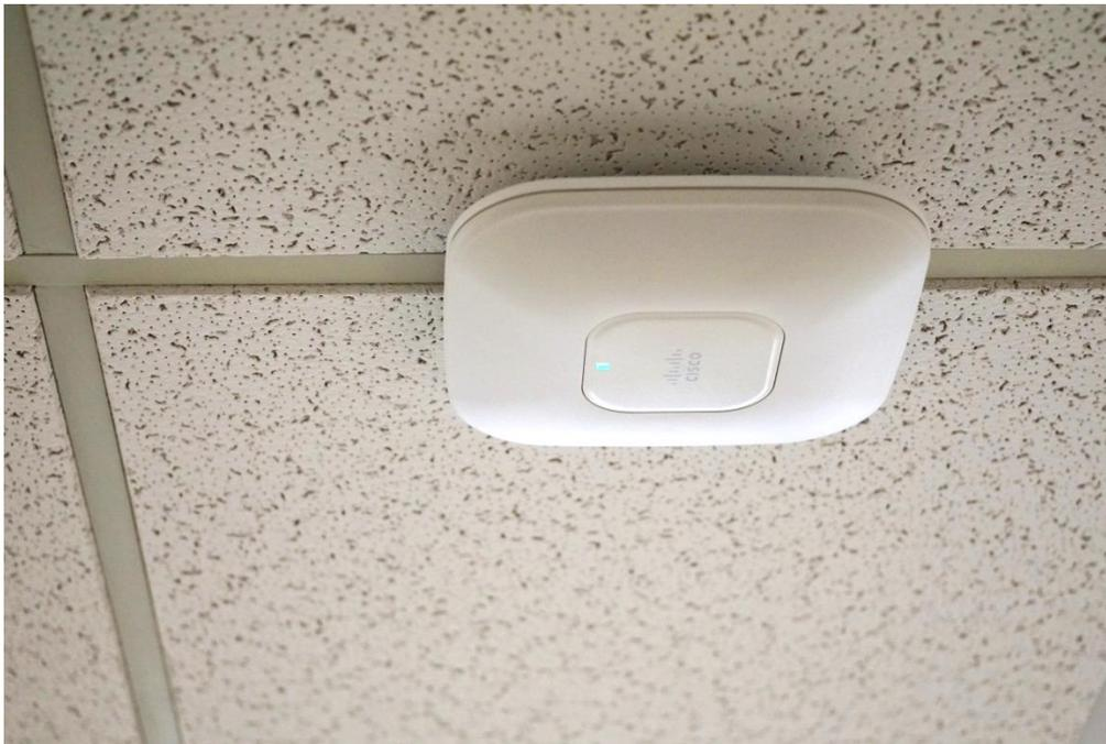
**A/P mounted on suspended ceiling T-Bar.**
