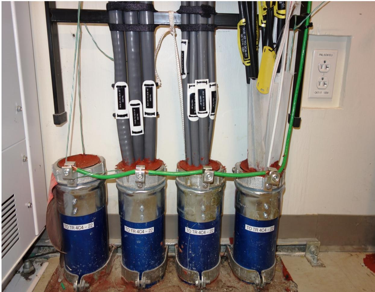
**Conduit stub-ups shown secured to floor-mounted strut.**
