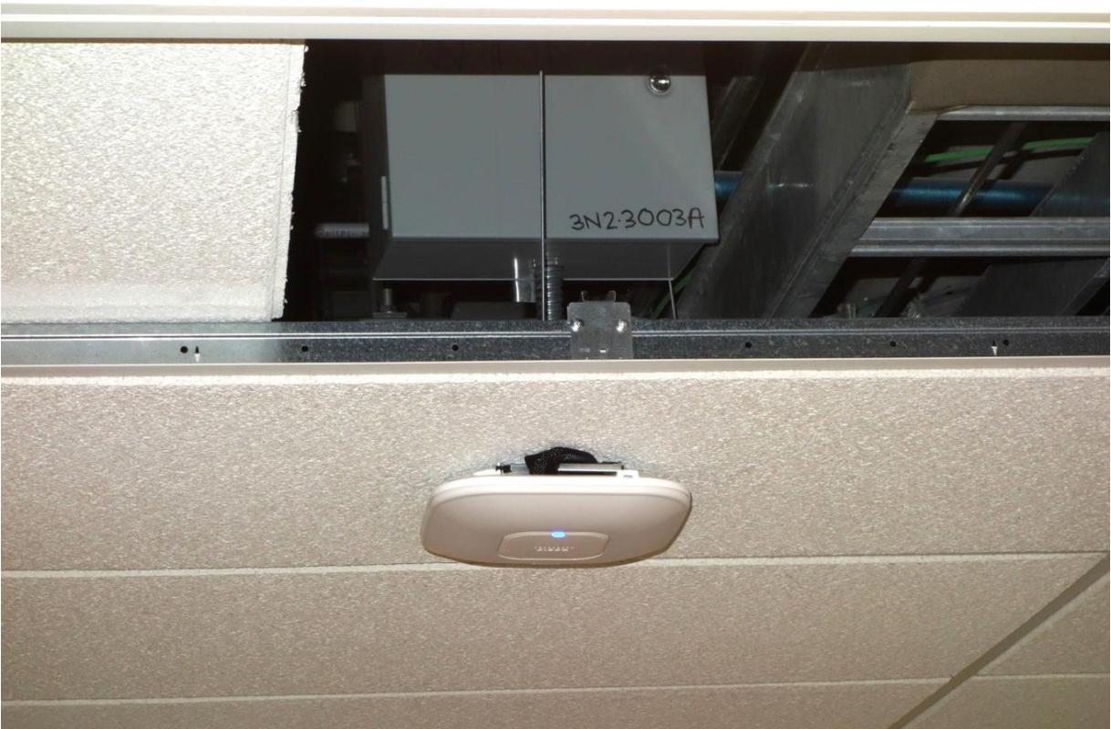
**A legacy A/P mounted in the center of a suspended ceiling tile prior to T-Bar mounting required.**
