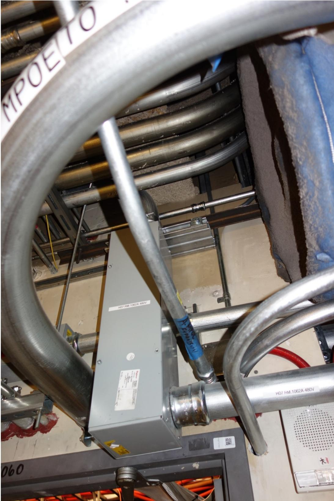
**Pull box for a 90-degree conduit direction change.**
