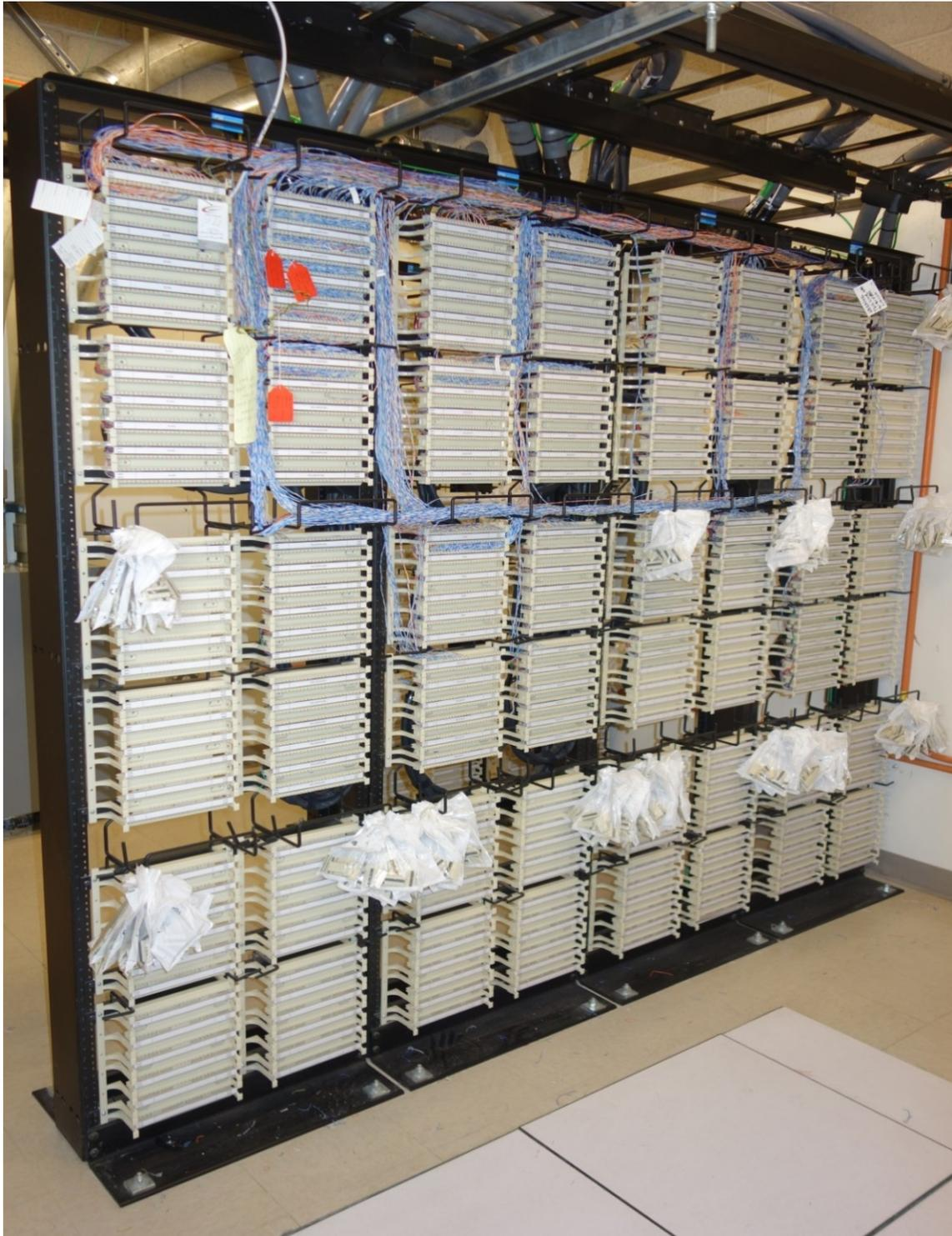
**Front View of an MPOE MDF shown with racks of 110 Blocks for Copper BD.**
