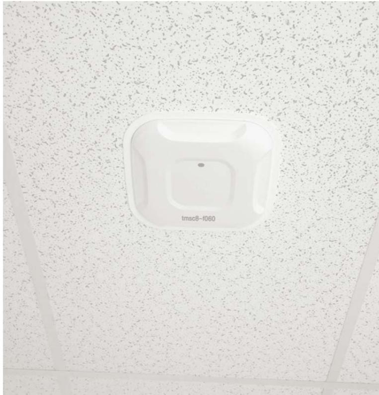
**A/P mounted within ceiling tile on the suspended ceiling T-Bar.**
