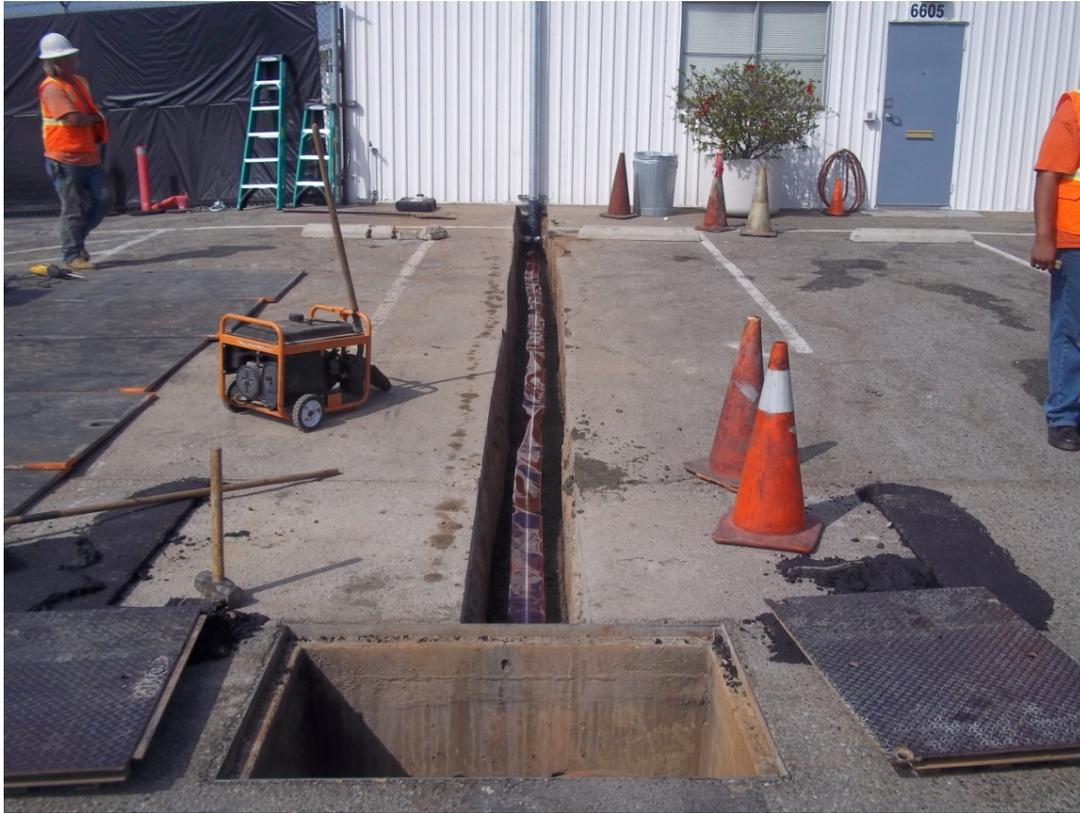
**Underground detectable identification tape installed.**
