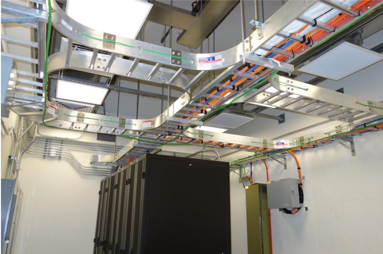
**Cable Tray that cannot reach perimeter walls due to obstructions shall have an additional lateral.**
