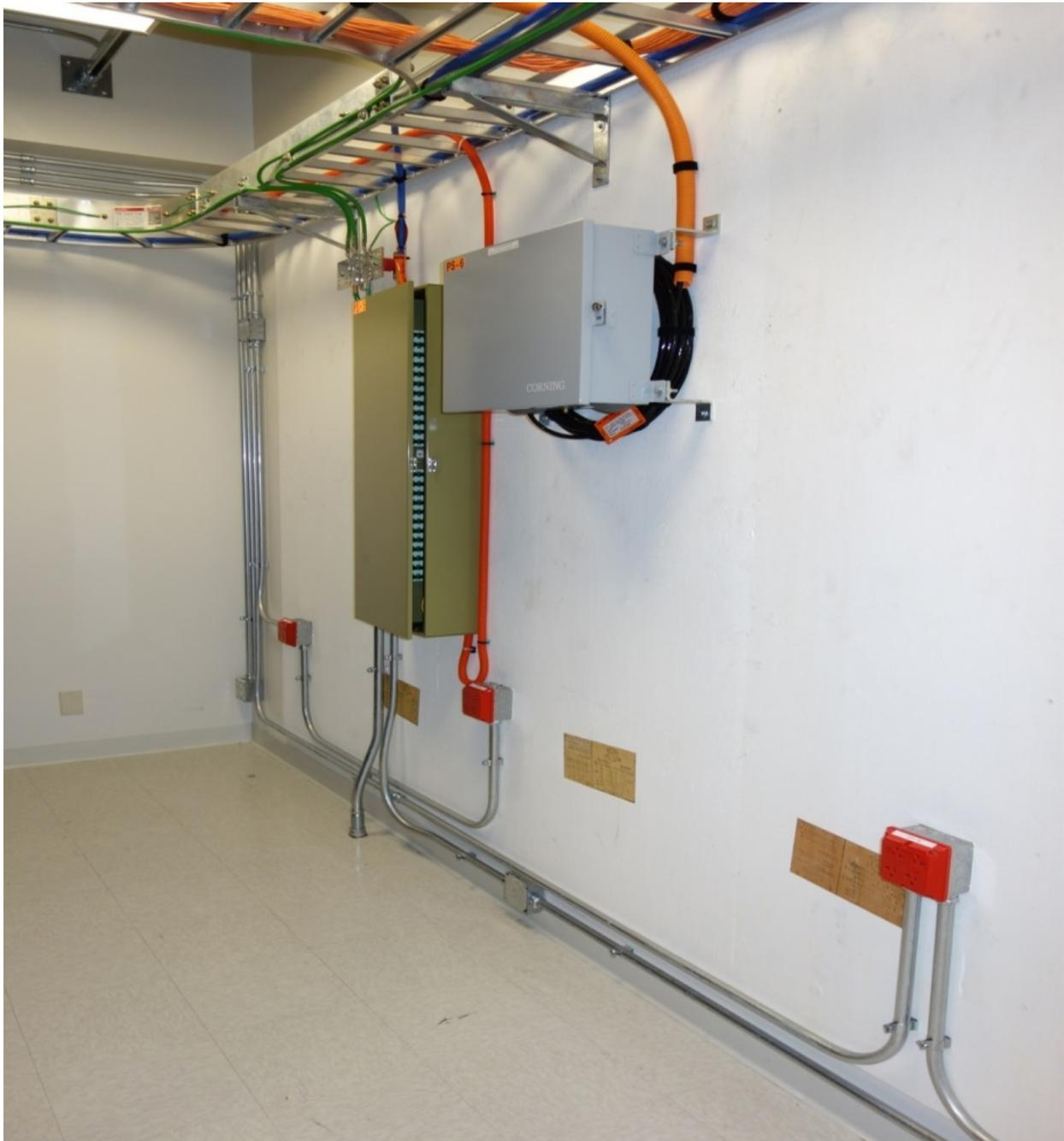
**Cable slack shall be coiled up behind wall-mount patch panels.**
