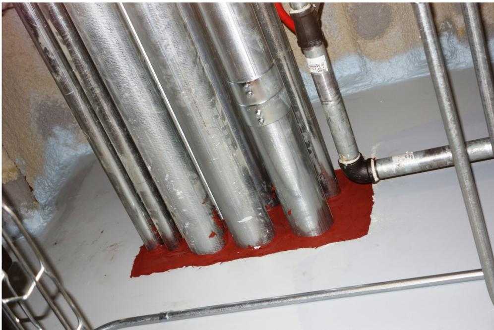
**Firestop putty around all individual conduits in a common wall entry.**
