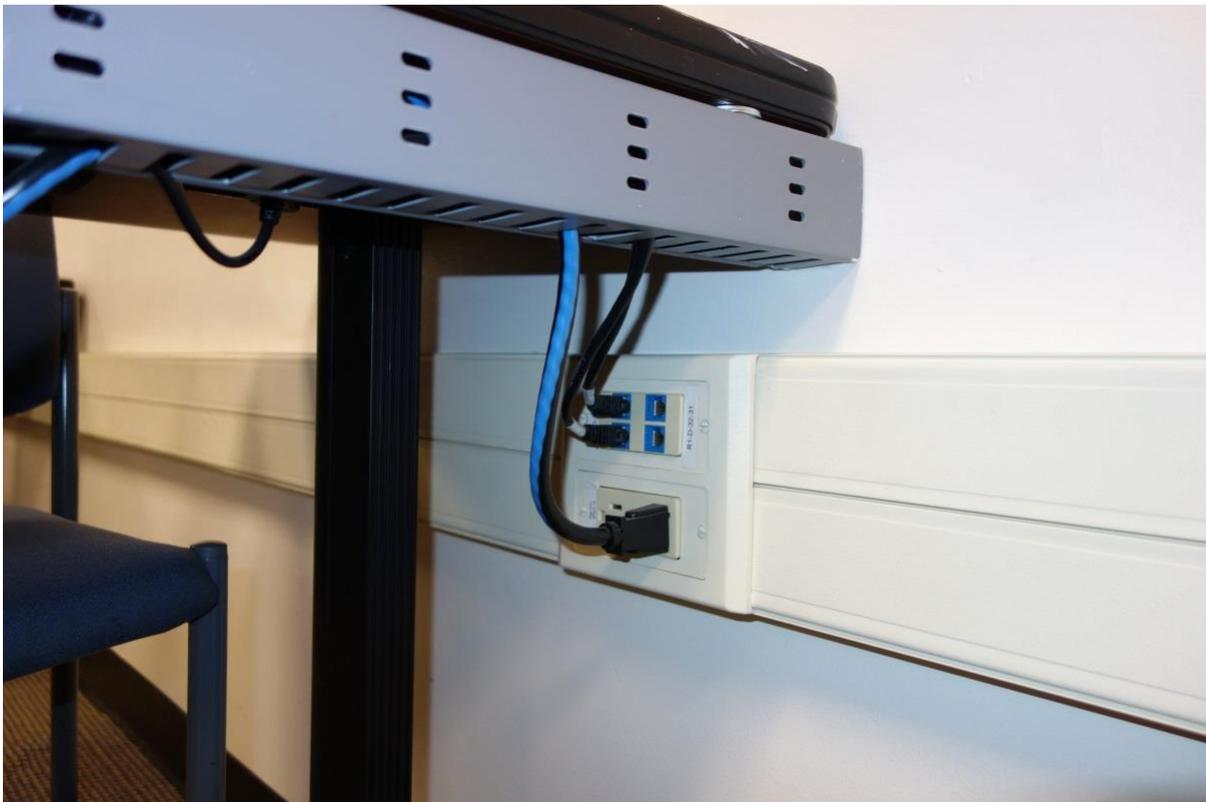
Surface-mount raceway is split to separate power and comm.
