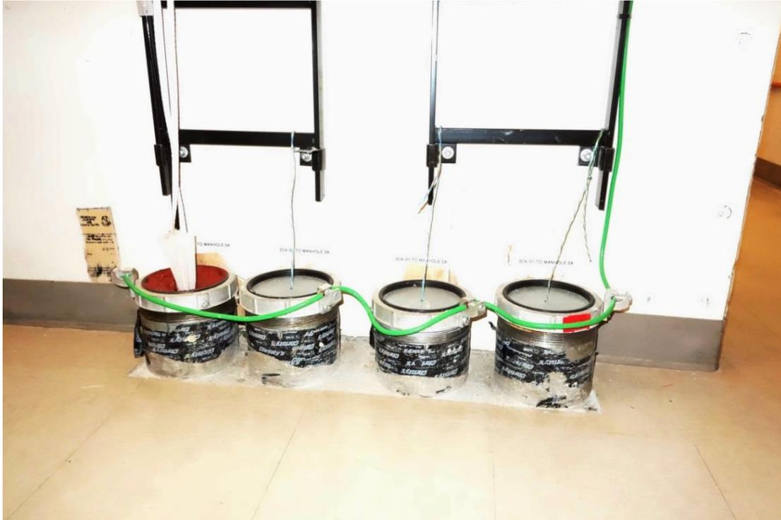
**Metal conduit bushings shown with grounding wires.**
