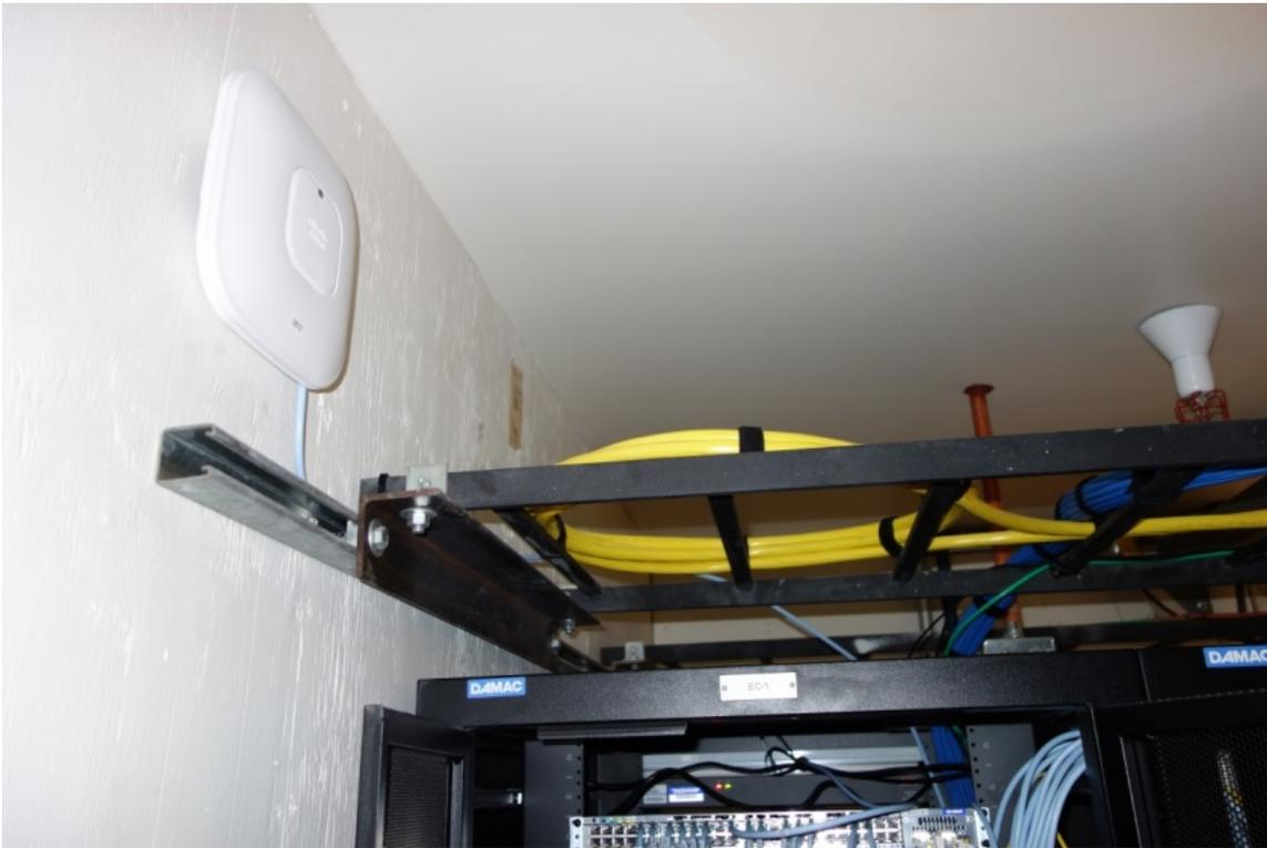
**A/P mounted in an IT Room on the side-wall.**
