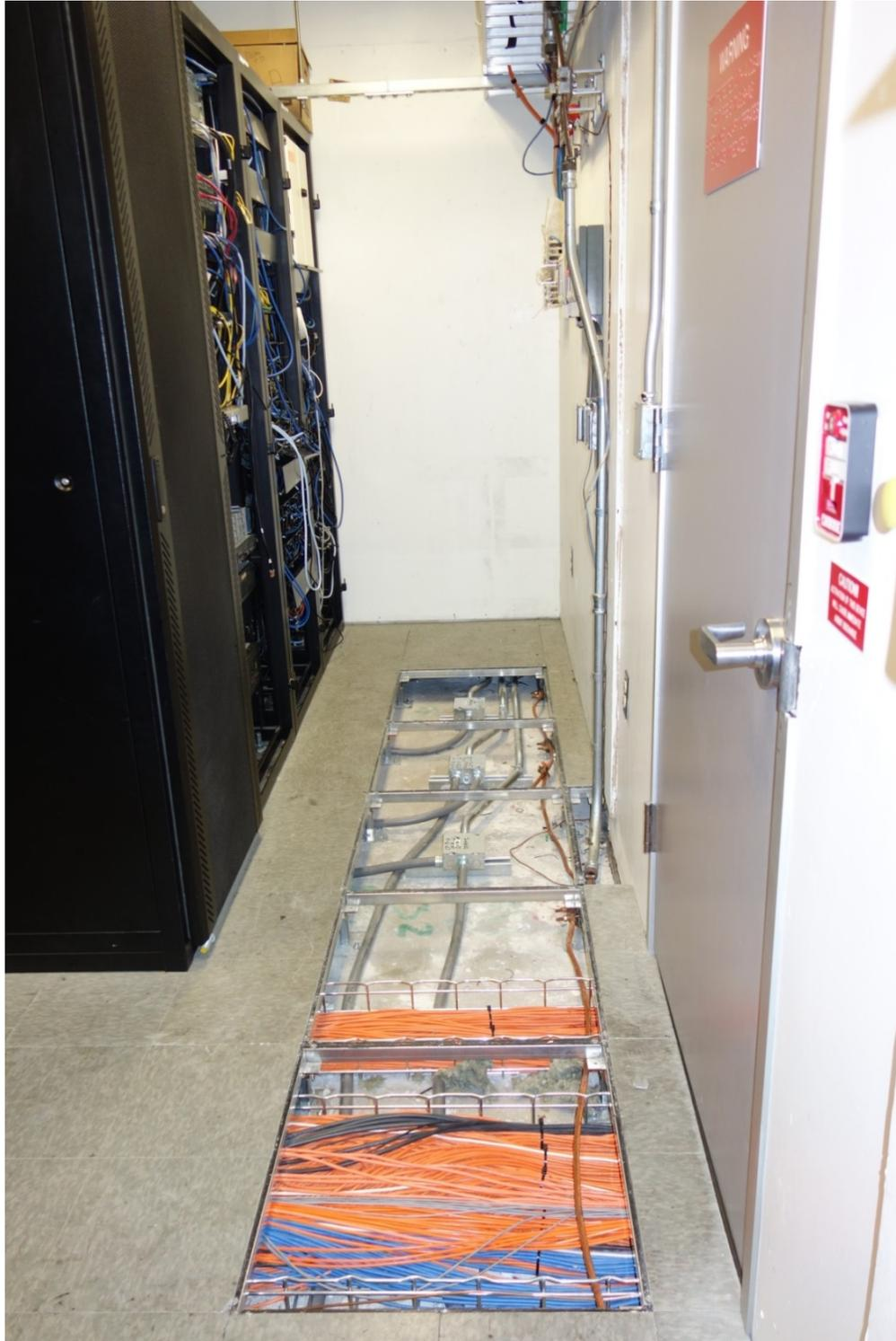
**Wire basket shown running under a raised access floor for horizontal cables in an IT Room.**
