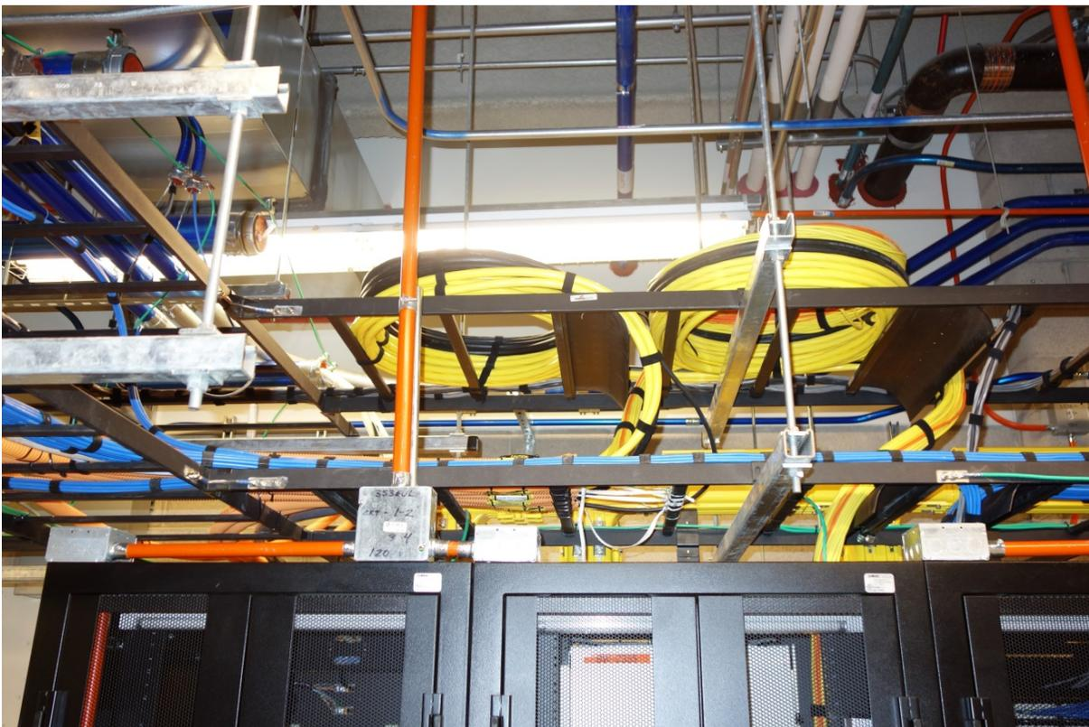
**One approved method of storing cable slack loop is to build a 2<sup>nd</sup> tier Ladder Rack.**
