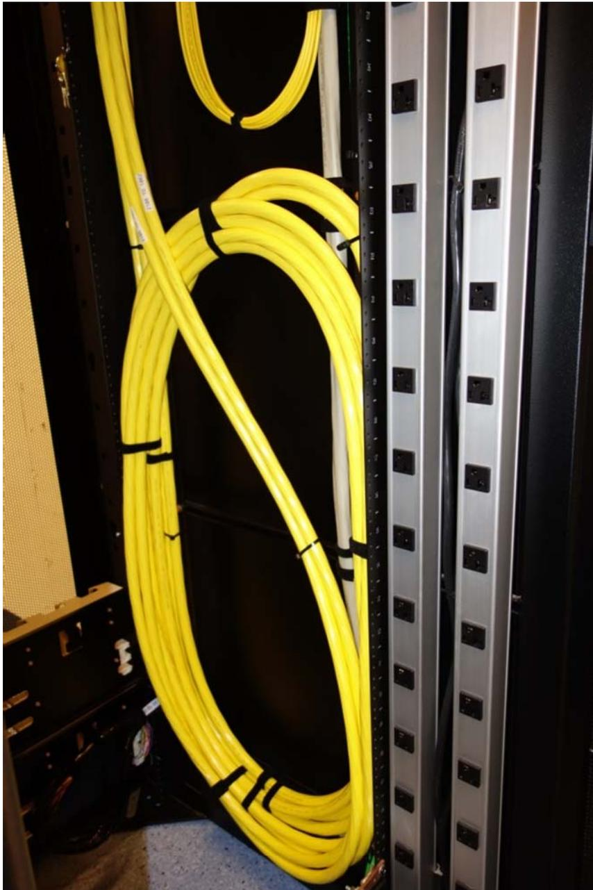
**If placed within a cabinet, cable slack shall go around the inside perimeter, not coiled up.**
