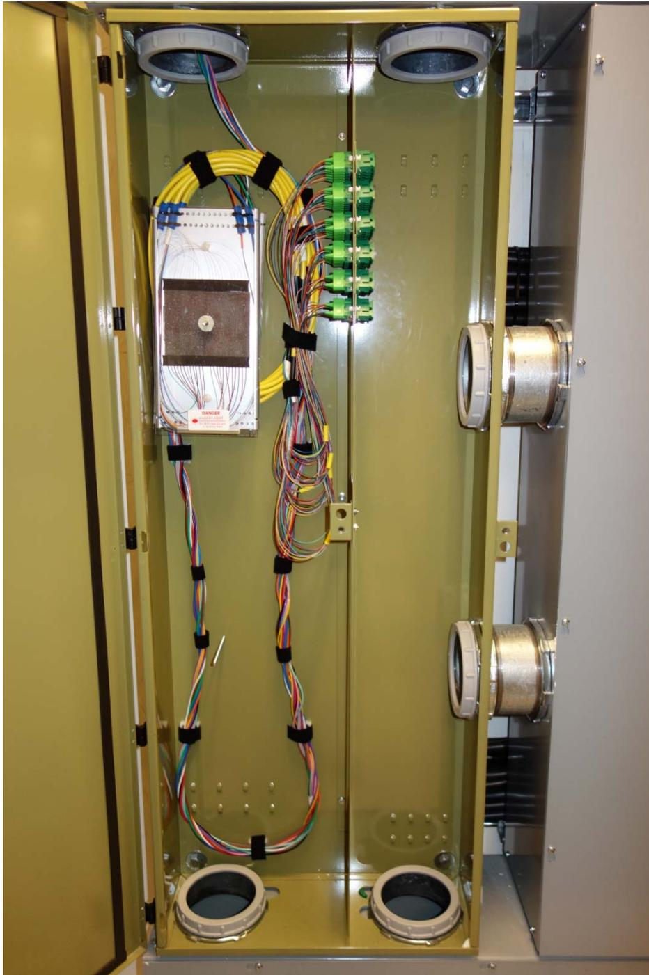
**Wall-mount FPP's shall have wireway and six 4-inch chase nipples installed as shown.**
