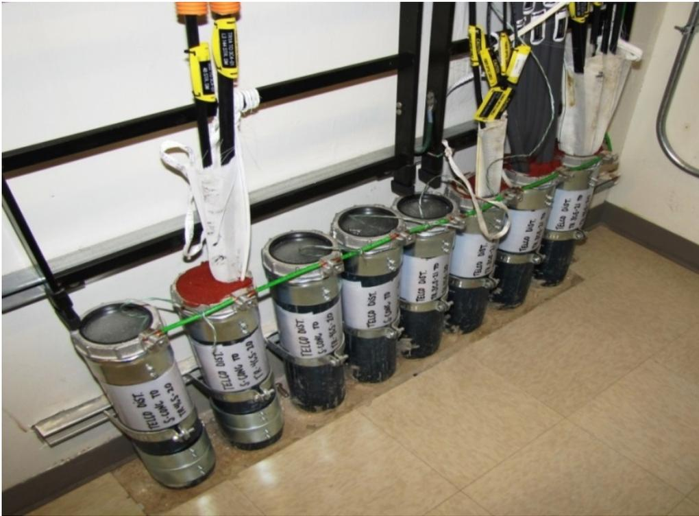
Conduit stub-ups shown secured to wall-mounted strut.
