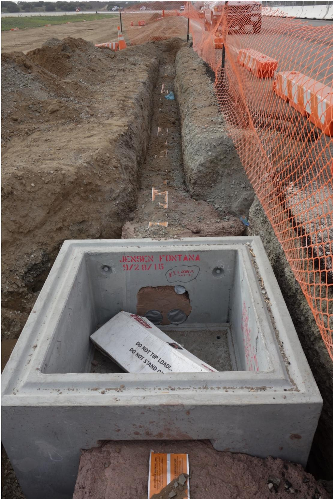
A ductbank using PVC concrete-encased conduits is shown with detectable I.D. tape.
