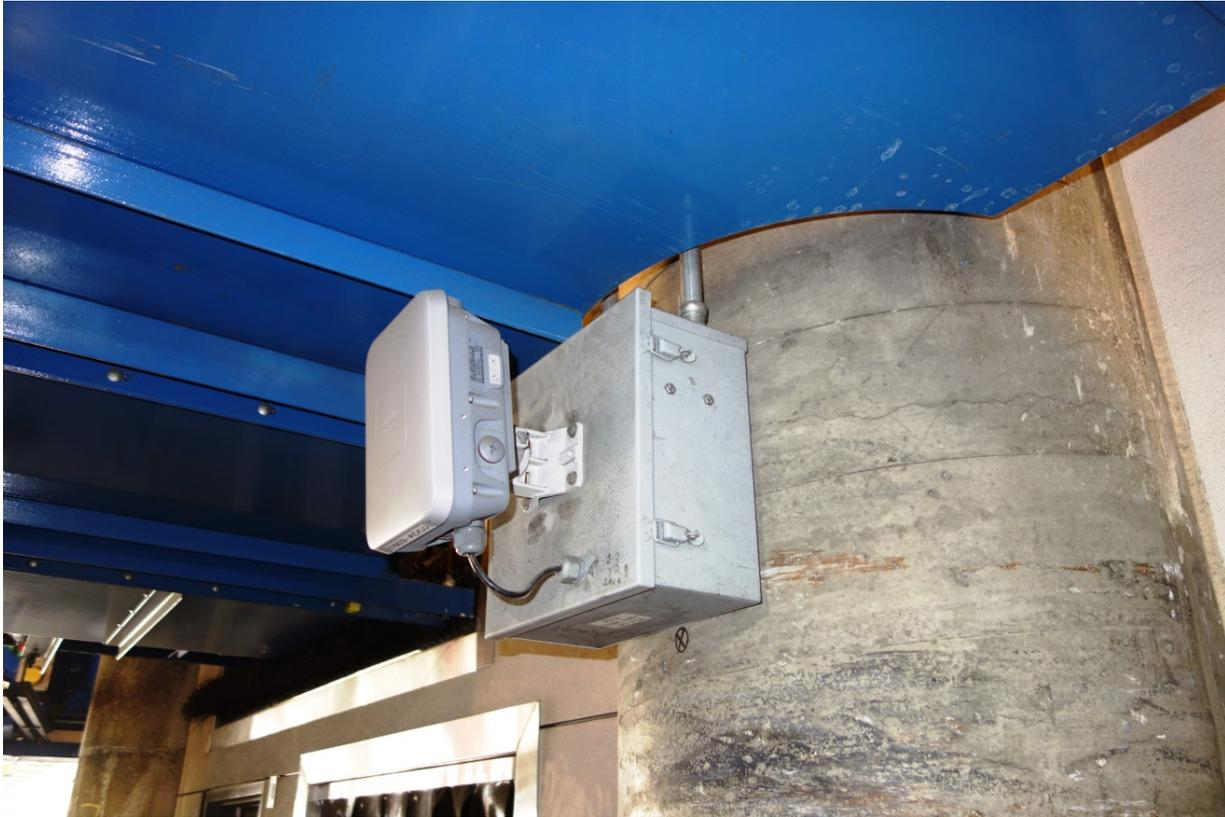
**An outdoor A/P is shown mounted on a support column.**
