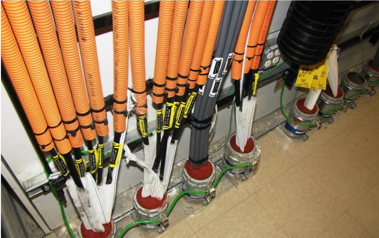
**The transition from HDPE innerduct to Maxcell fabric innerduct within conduits is shown.**
