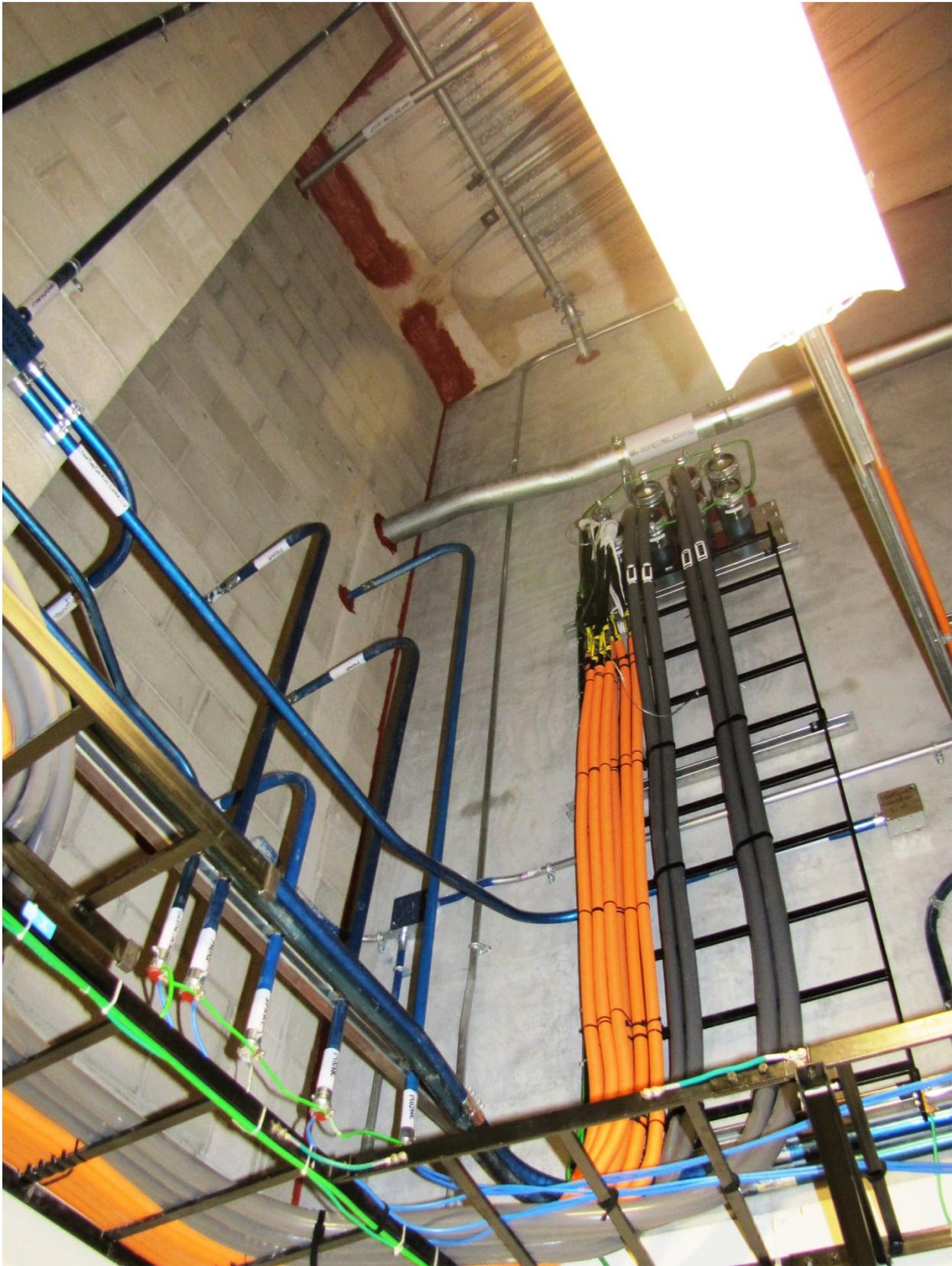
**In IT Rooms, vertical Ladder Rack is required to secure cables for conduits that don't reach within 12-inches of the cable tray or ladder rack.**
