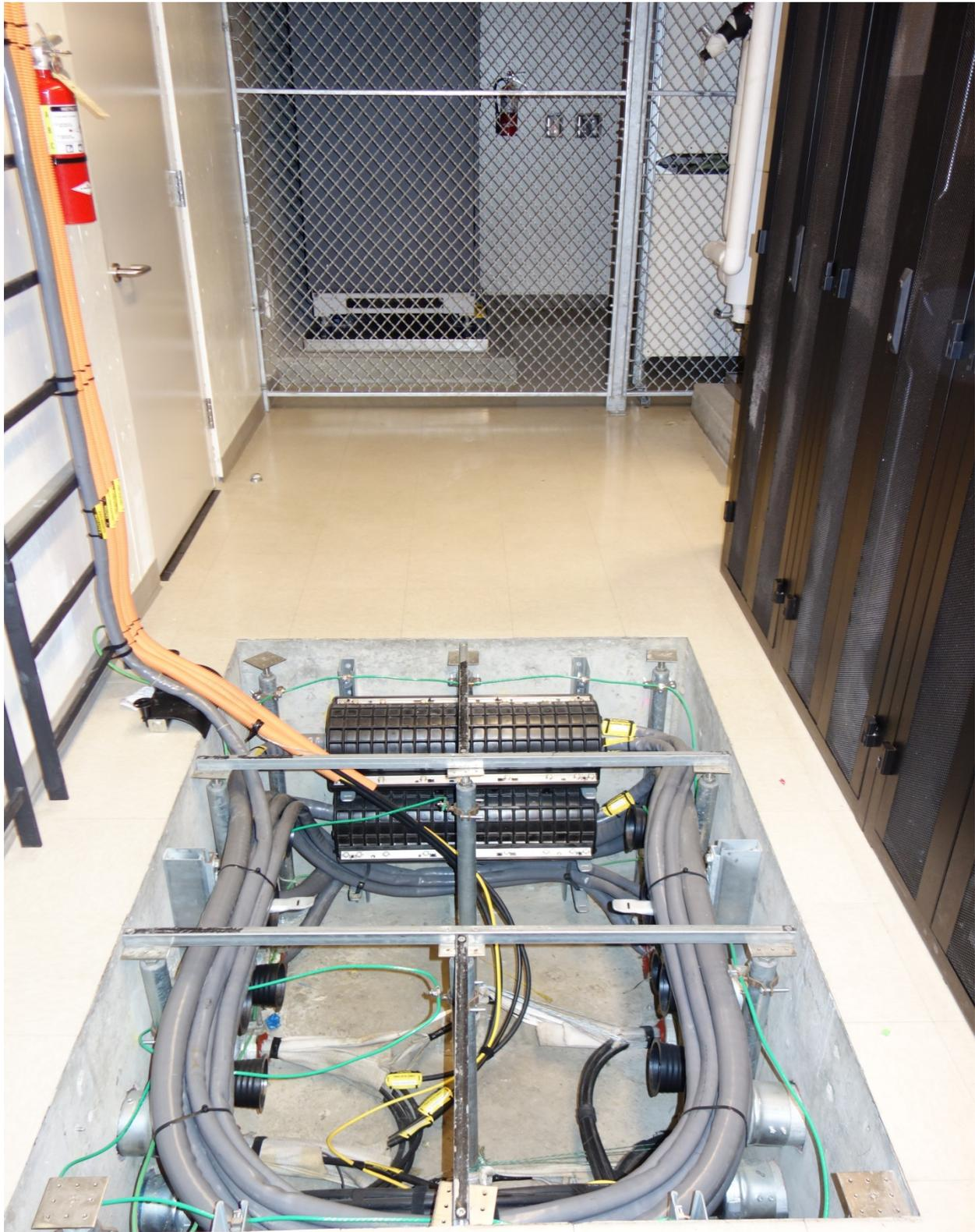
**Conduit wells shall be nest to the IT Room wall so that cables are not a trip hazard as shown here.**
