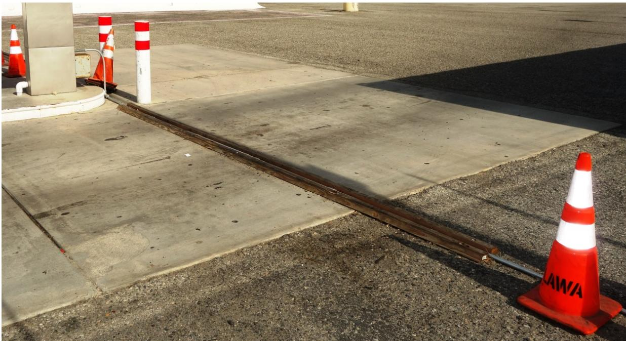
**Conduit-protector at fuel pump protecting conduit.**
