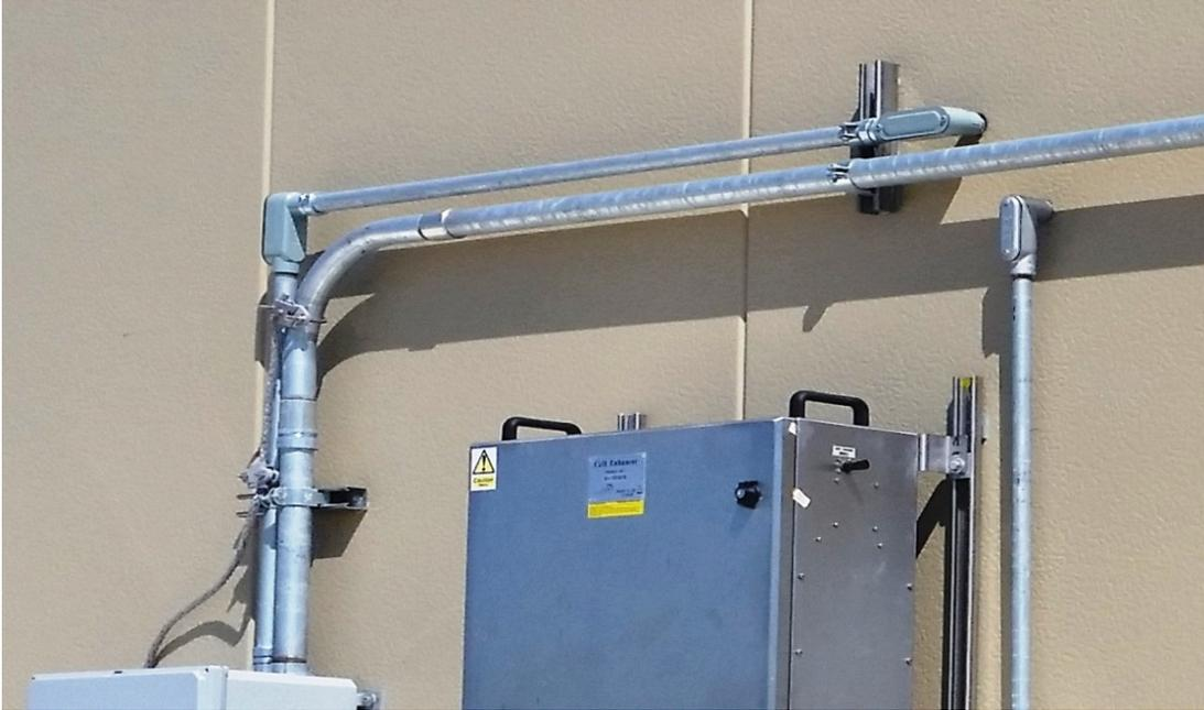
**Conduit bodies/condulets used for copper cables.**
