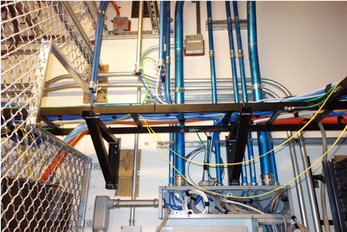
**Wireway is shown with cable slack loops for an IT system.**
