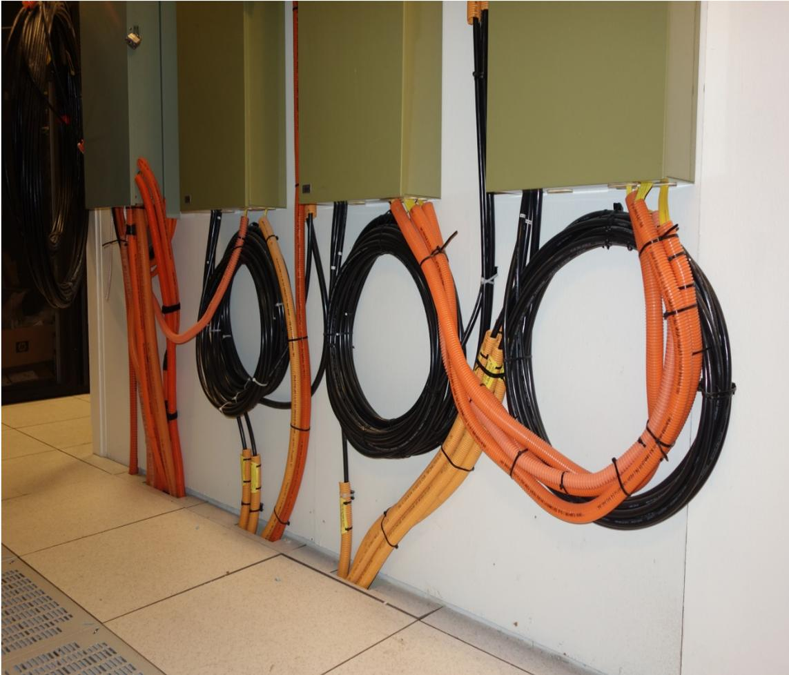
**Legacy fiber slack previously mounted on walls is not coiled up behind patch panels.**
