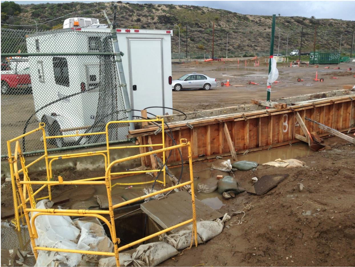
**A sample of a required safety barricade surrounding a Hand Hole entrance prior to splicing.**
