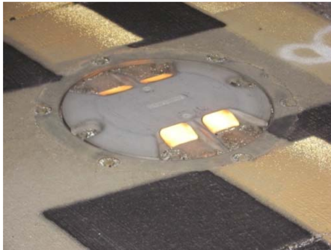
Flush-mounted Runway Light Fixture
