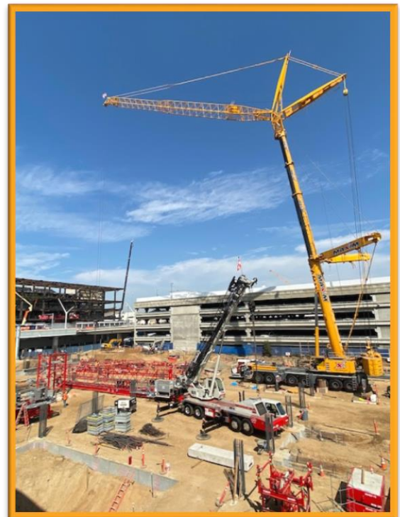
In-progress shot of future West CTA tower crane (red) being built
