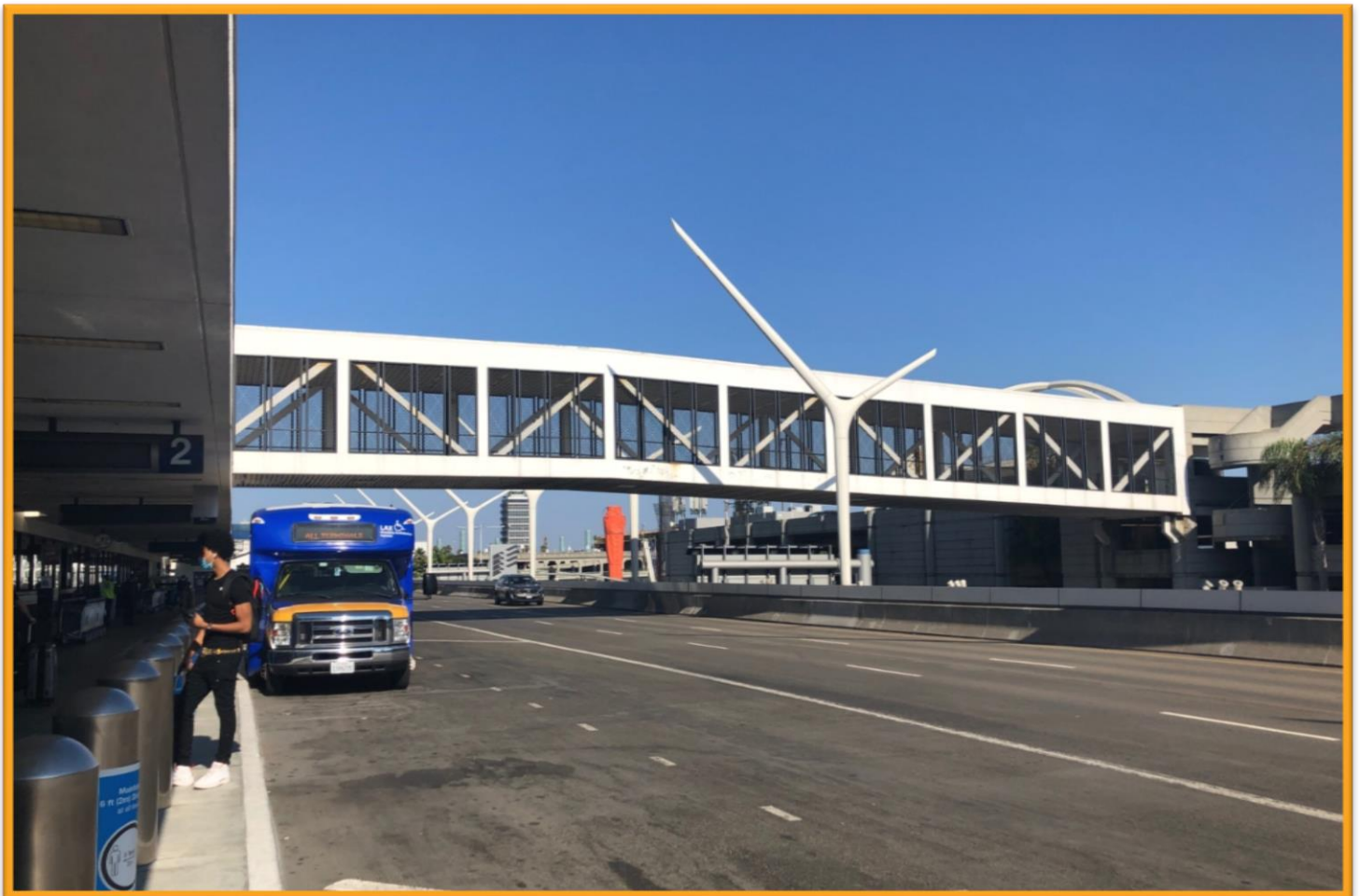
Pedestrian Bridge between Terminal 2 and Parking Structure 2A, pictured from the Departures Level roadway looking east
